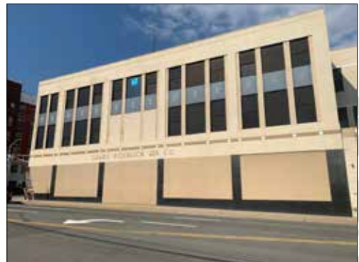
Figure 7.2: Three (3) story historic facade of Sears Roebuck and Company building on E. Anderson Street
