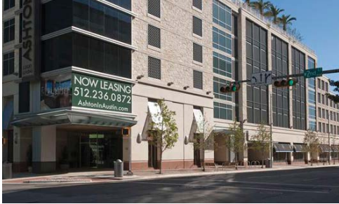
Figure 3.16: Screened parking garage
