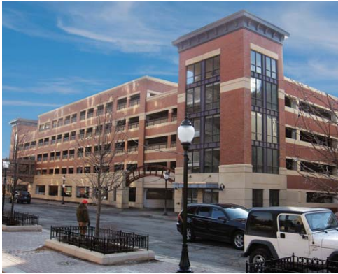
Figure 3.17: Screened parking garage
