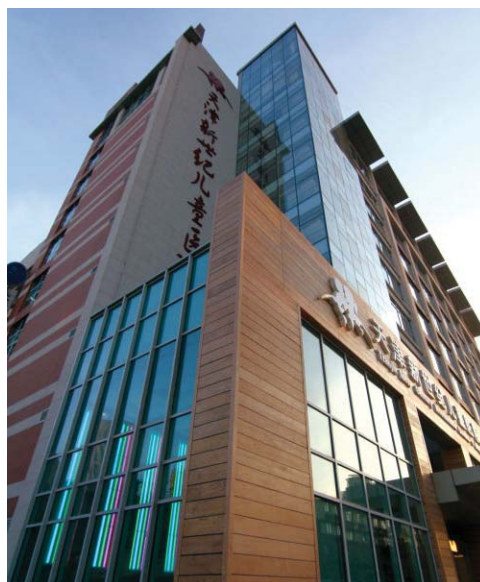
Figure 3.14: Exterior wood paneling
