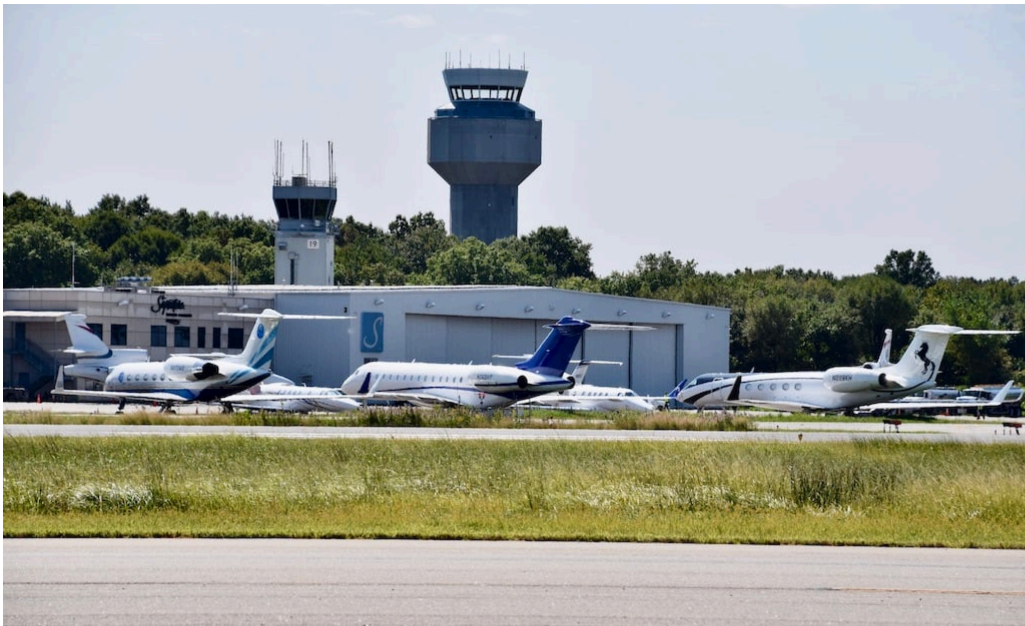
The FAA's new ATC tower overlooks the existing tower at Teterboro Airport. Credit: Bill Carey
