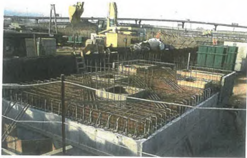
Above, the Vortechs® cast-in-place System during construction. Each of the roof slabs for the cast-in-place units include a steel cross beam to help meet the loading specifications.
